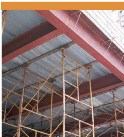
LESSER SCAFFOLDING REQUIREMENT
